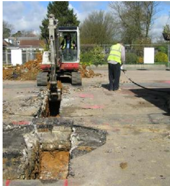
Norman Herridge scooping up the soil under the original tarmac & concrete to reach the depth of the new building's foundations, whilst Kevin uses the percussion hammer on more concrete.
