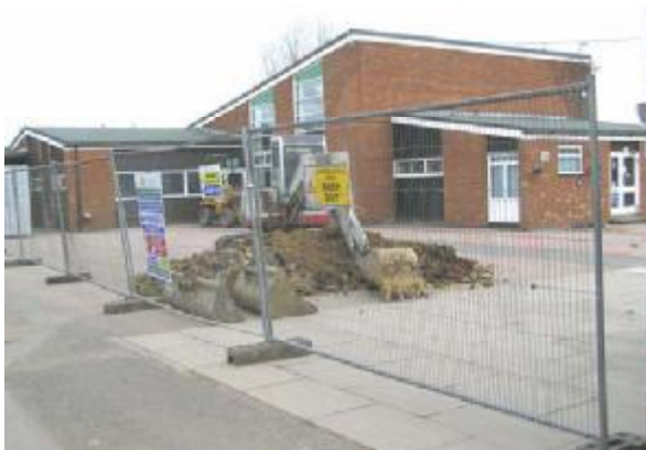
The original space between the two buildings
