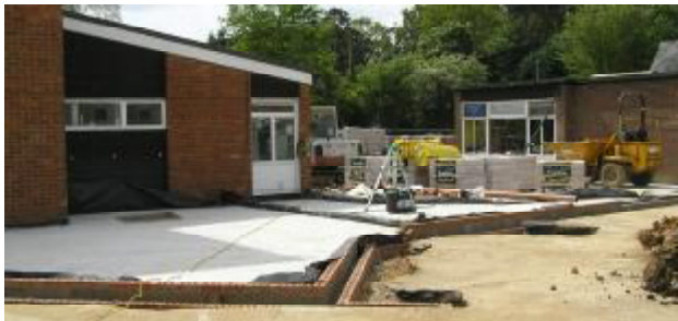
▲ The floor slab cast in concrete, showing the overall floor plan ▼
