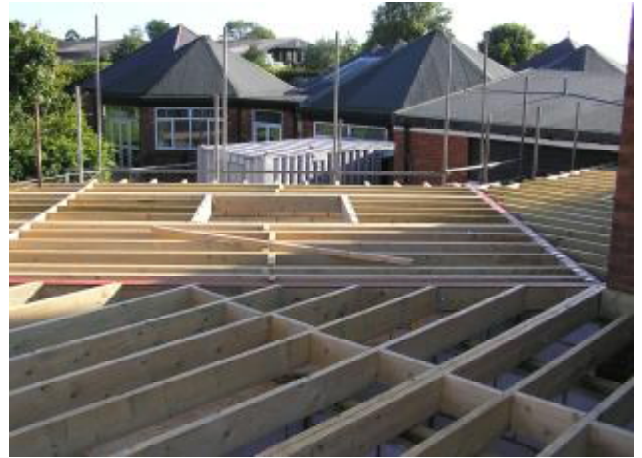
With the Glulam Beams in position, the roof structure takes shape ▼
