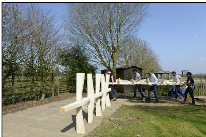
Carrying the side wall into place
